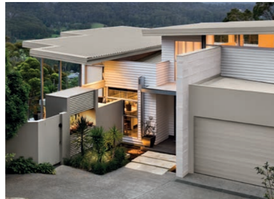
• Roofing and garage door | COLORBOND® steel Dune® in a Classic finish.
